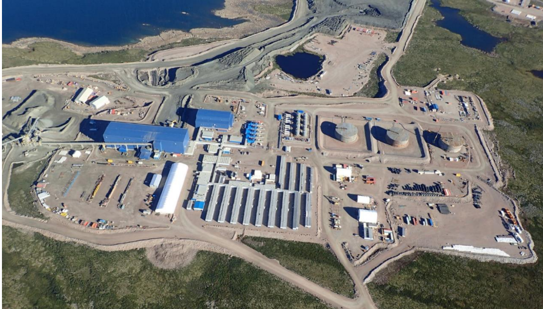
Figure 1-4: Gahcho Kué Mine Site Q3 2017
