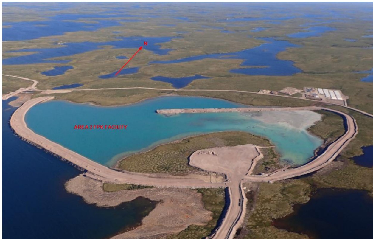
Figure 17-4: Area 2 Fine Processed Kimberlite Facility Q3 2017
