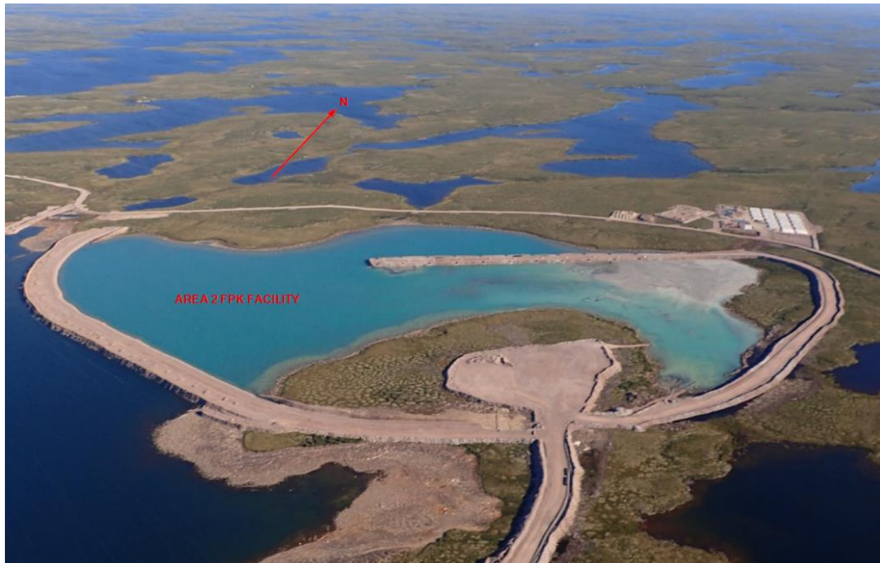
Figure 17-4: Area 2 Fine Processed Kimberlite Facility Q3 2017
