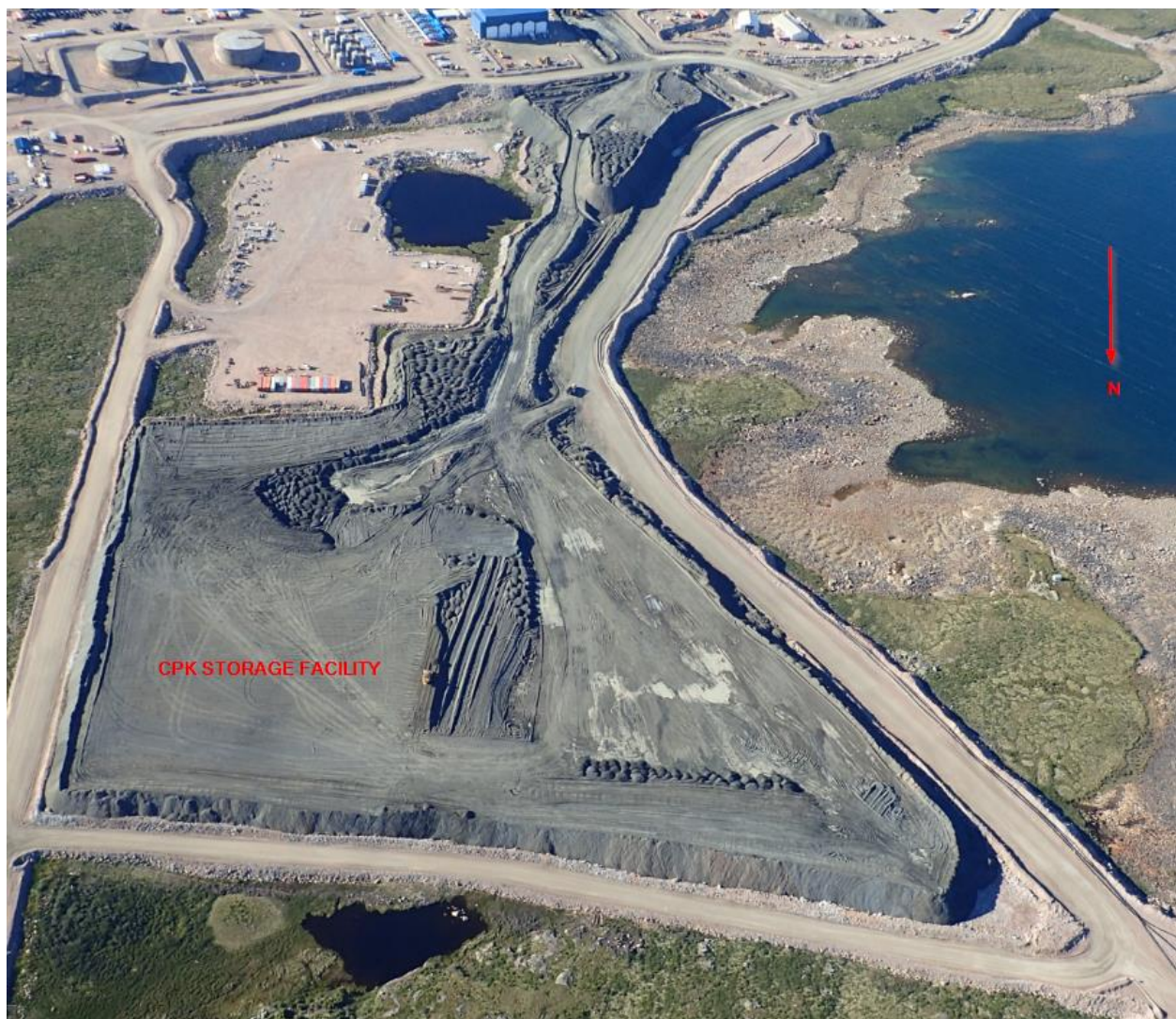
Figure 17-3: Coarse Processed Kimberlite Pile Q3 2017
